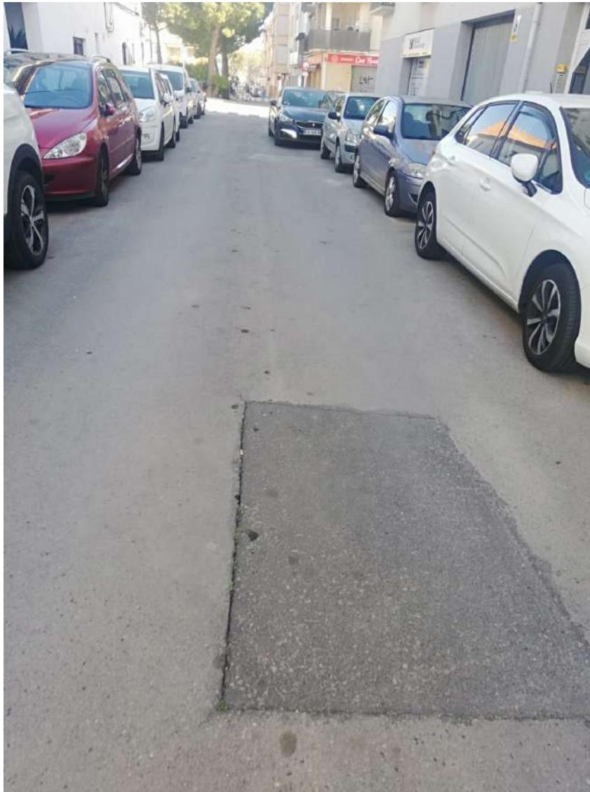
Vista general carrer Torreta
