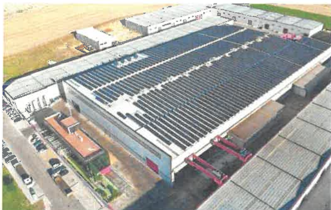
Nau Tecade, Sevilla – 990,12 kWp
